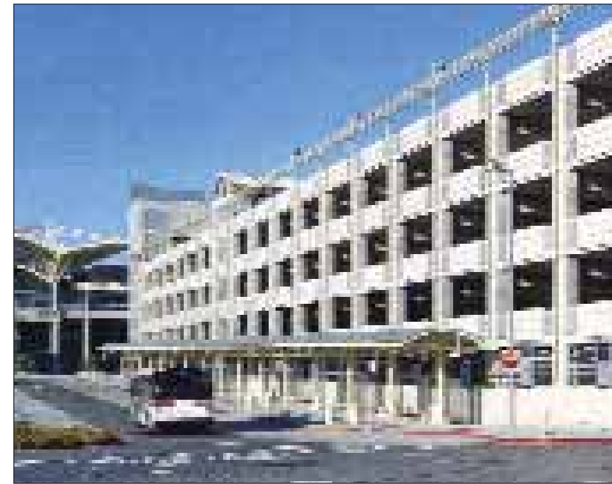
MILLBRAE MULTI-MODAL STATION PARKING STRUCTURE, SAN FRANCISCO, CALIFORNIA
